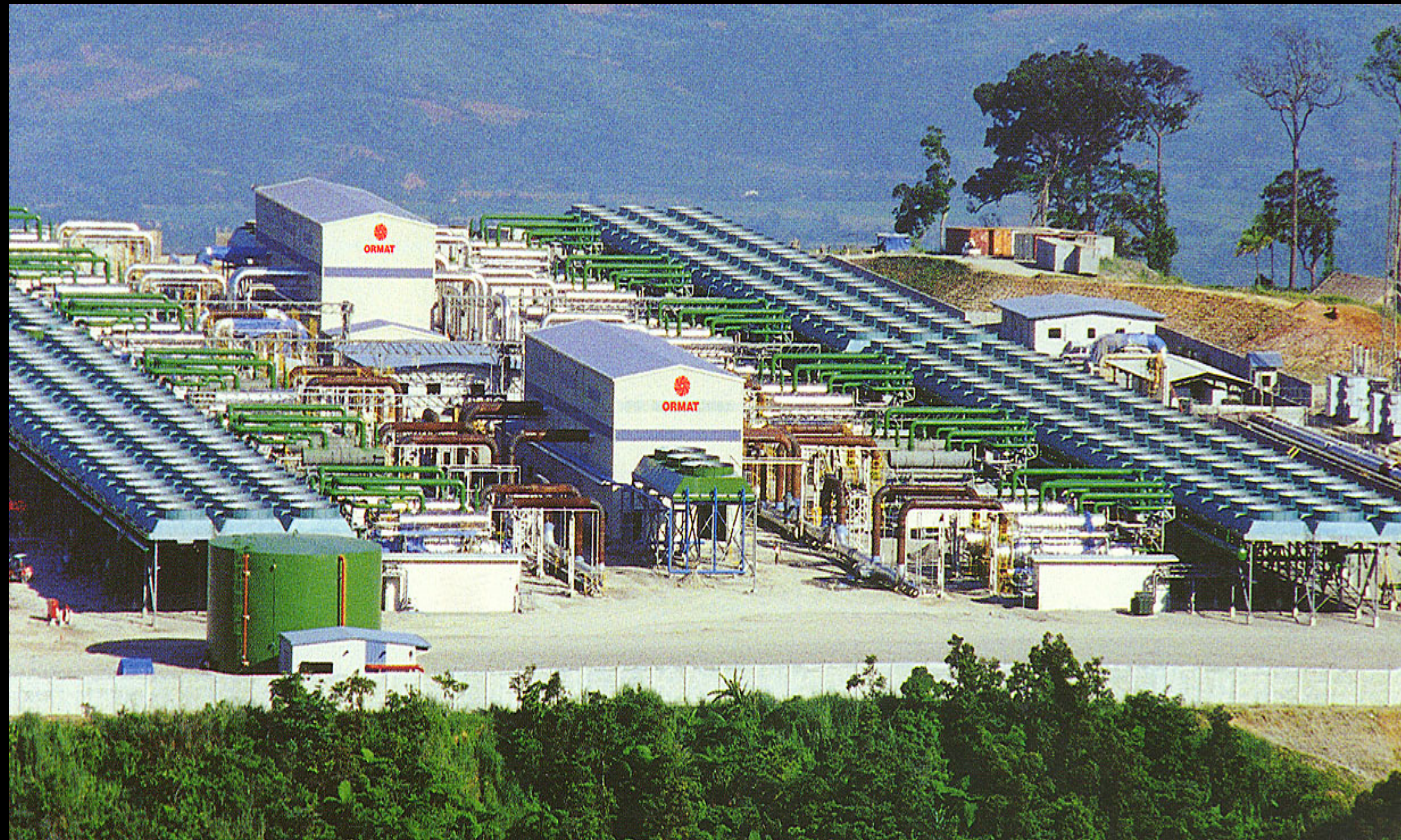
Upper Mahiao plant, the Philippines
