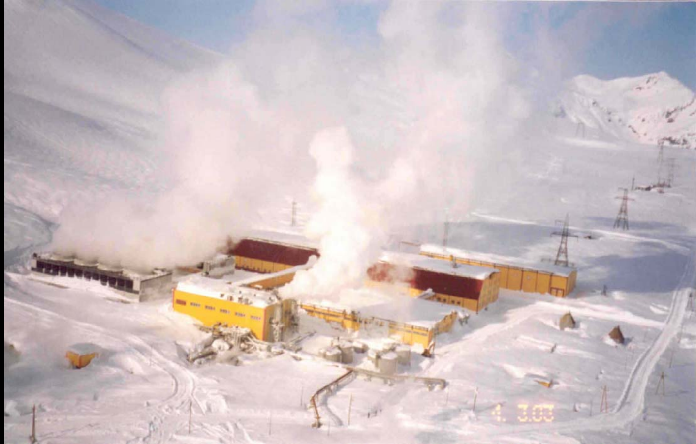
Mutnovskiy 50 MWe Power Plant, Russia,
