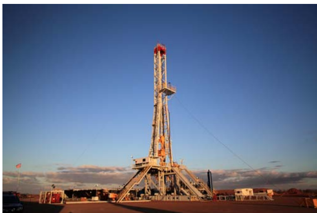
Drilling Begins at Paralana
